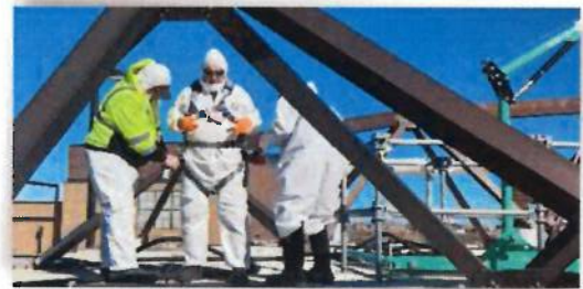
Employees suit up to enter and manually remove wipes and rags from a gravity thickener at the NTP.
