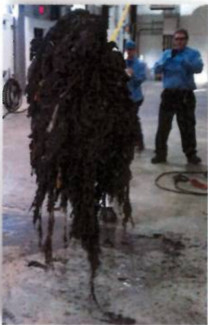
Wipes mix with rags and debris to clog pipes and equipment at the Robert W. Hite Treatment Facility (left) and Northern Treatment Plant (NTP) (right).
