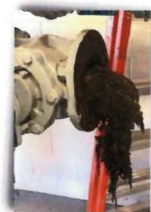
Wipes mix with rags and debris to clog pipes and equipment at the Robert W. Hite Treatment Facility (left) and Northern Treatment Plant (NTP) (right).
