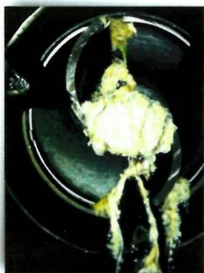
Wipes clog pipes (left) and equipment such as pumps (right), requiring regular, manual removal of wipes mixed with rags at Metro's Northern Treatment Plant (photo top of page).
