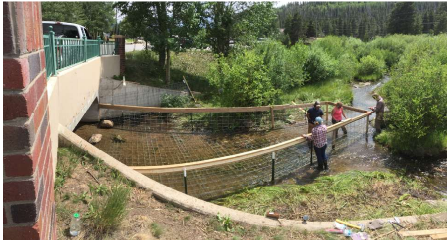
Figure B-5. A large re-enforced Keystone fence installed by EcoMetrics has been effective at keeping beavers from damming this large box culvert. Photo by Mark Beardsley.
