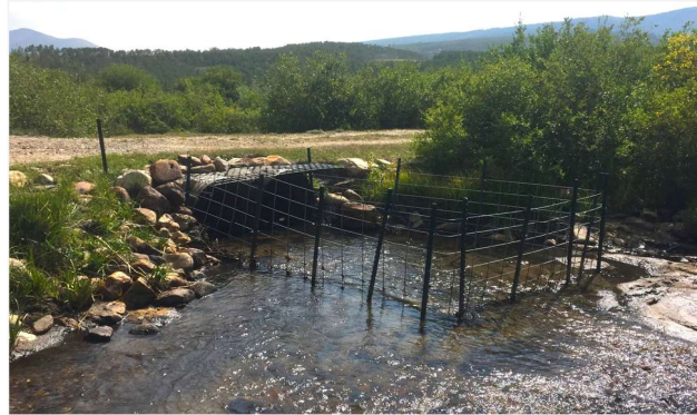
Figure B-4. A keystone fence installed by EcoMetrics to protect a road culvert on a tributary of the South Platte river in Park County. Photo by Mark Beardsley.
