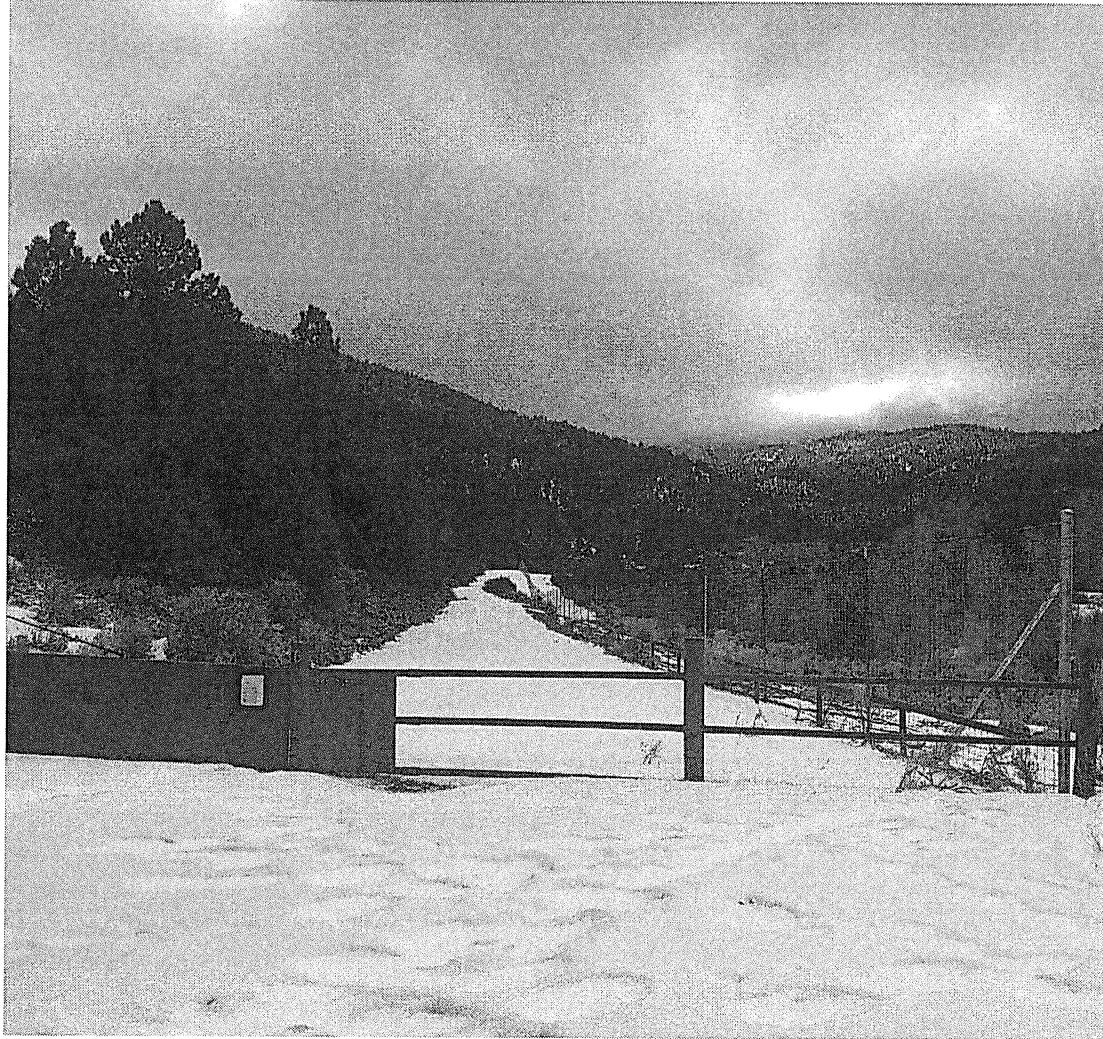
New Fence San Francisco Creek
