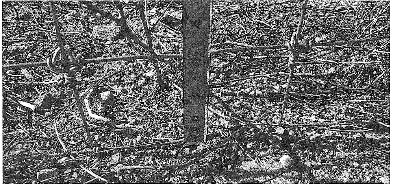
Photograph of Cielo Vista Ranch fence showing dimensions of fence openings of the fence.
