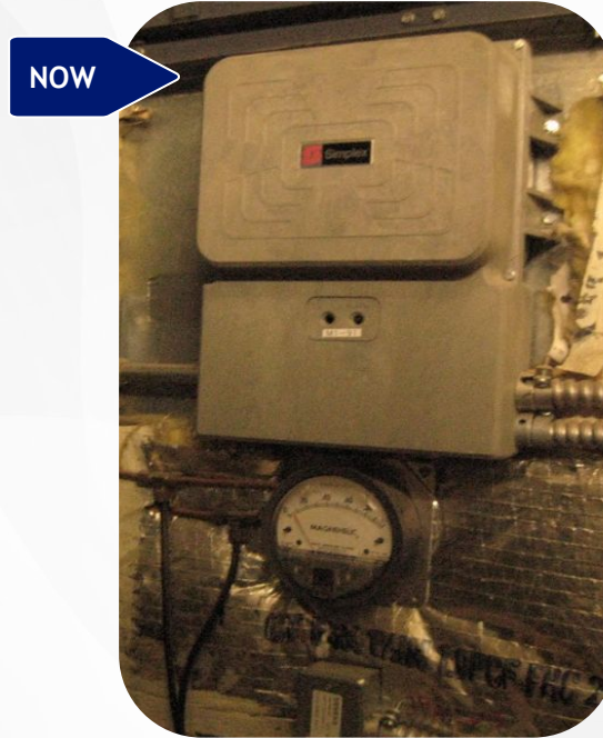
Fire Alarm Device Upgrade (MapNet to IdNet)
