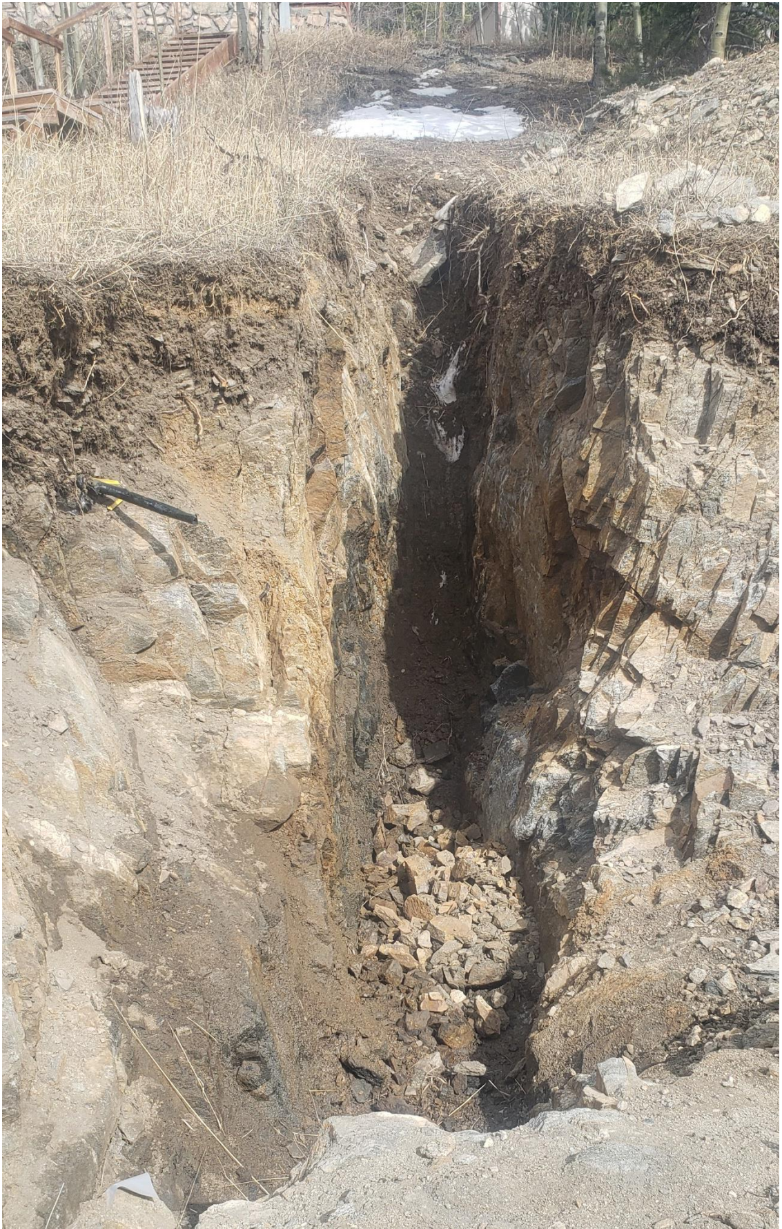
Re-Routing Water Lines requires trenching through rock
