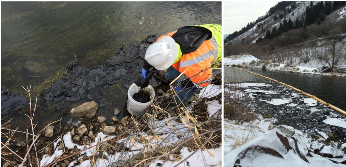
Provo River spill. EPA captions read: (L) “Collecting oil along the bank by the spill site. Much of the congealed oil can be removed by hand;” (R) “Snow-covered crude oil successfully collected by the boom at the Diversion [Dam].”
