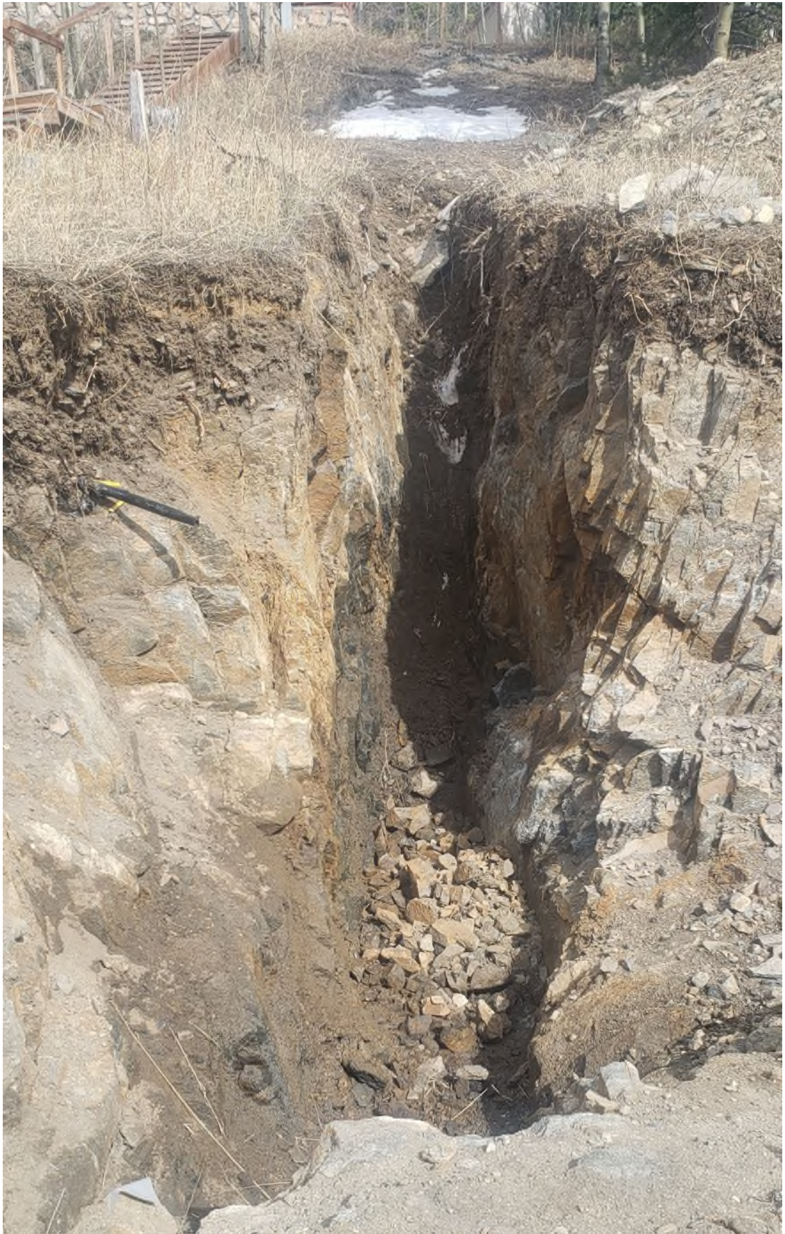
Re-Routing Water Lines requires trenching through rock
