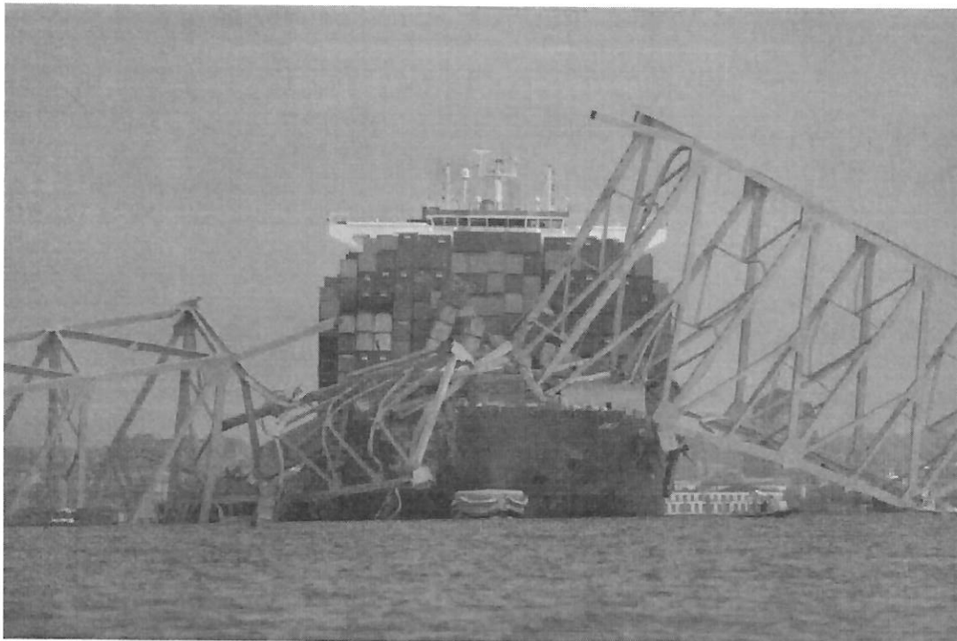
Photos: Baltimore's Francis Scott Key Bridge collapse ( msn.com )
