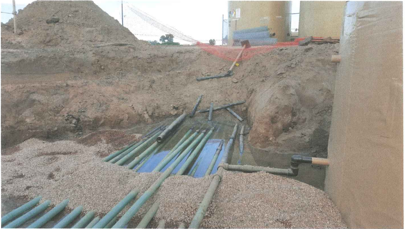
Gas Well Company Tring to do some repair work. They had to bring in a pump in order to get the water down low enough to do the repair work.
