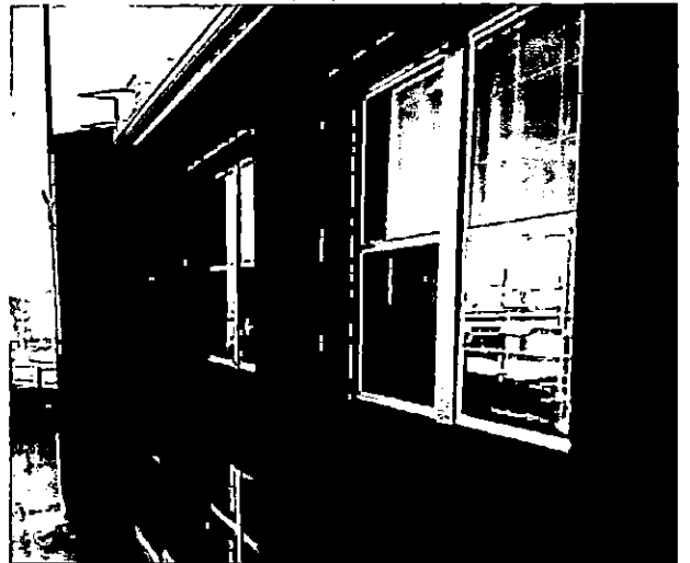
North side windows, after
