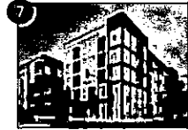
ALTA CITY HOUSE (2015) 5 Story, 281 Apartments
