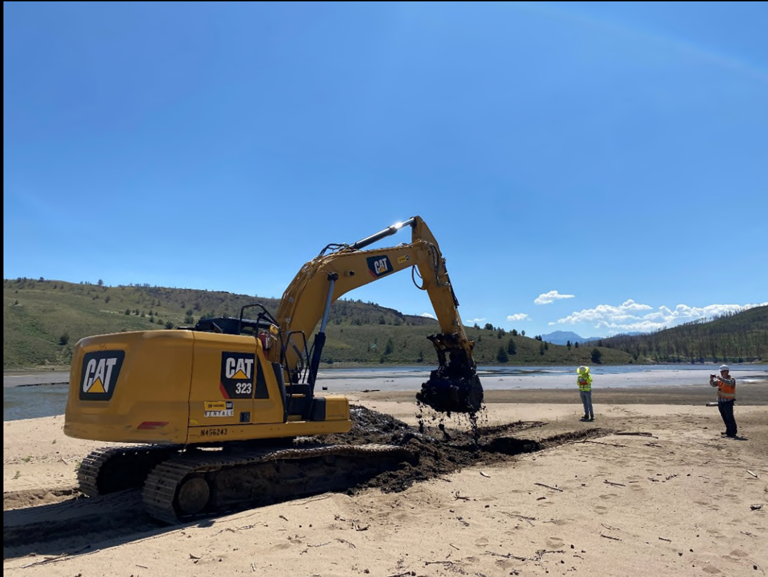
Test pits at Willow Creek Reservoir Berm location for geotechnical investigation 7/22
