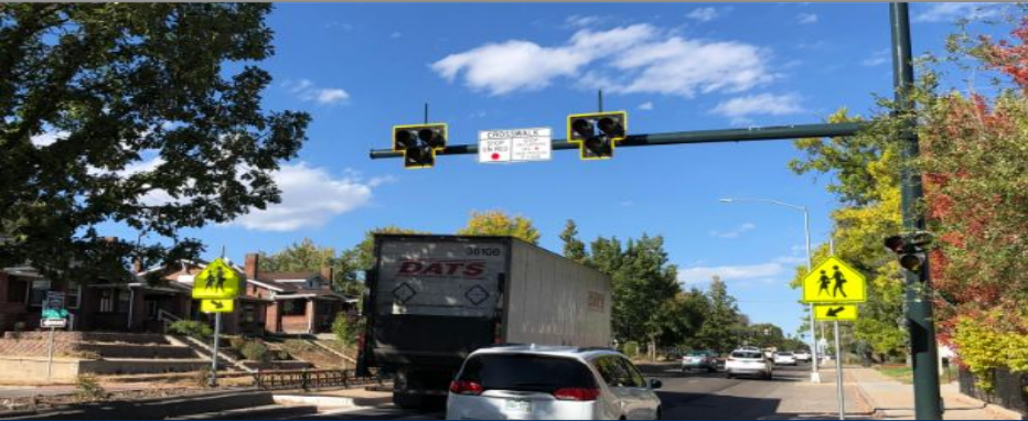
Region 1 - Federal and 42nd - Pedestrian (Ped) Actuated High-Intensity Activated CrossWALK (HAWK) Signal
