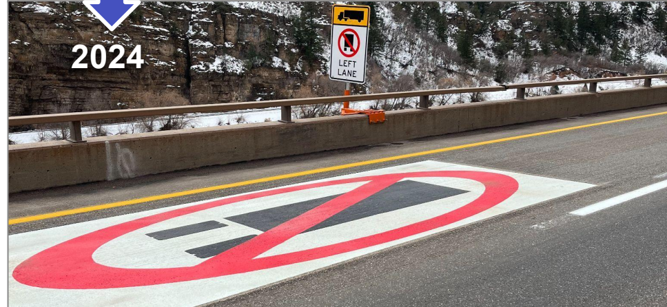
Region 3 - Glenwood Canyon Symbolic Sign Upgrades
