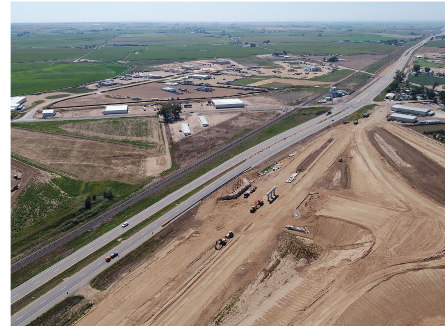
Grade separation project in progress – Weld County Road 44 at US Highway 85
