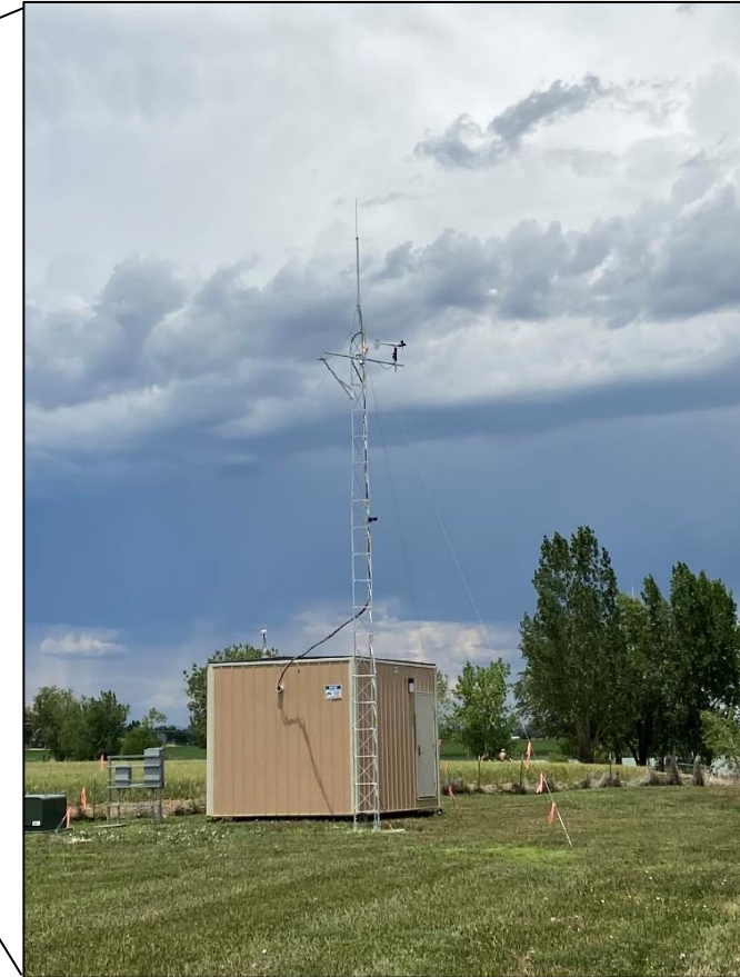
Union Reservoir Station
