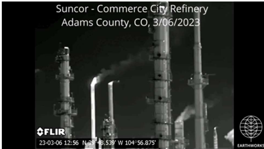
OGI video captured by Earthworks shows plume of pollution (invisible methane and VOCs) from major source on the Suncor refinery
