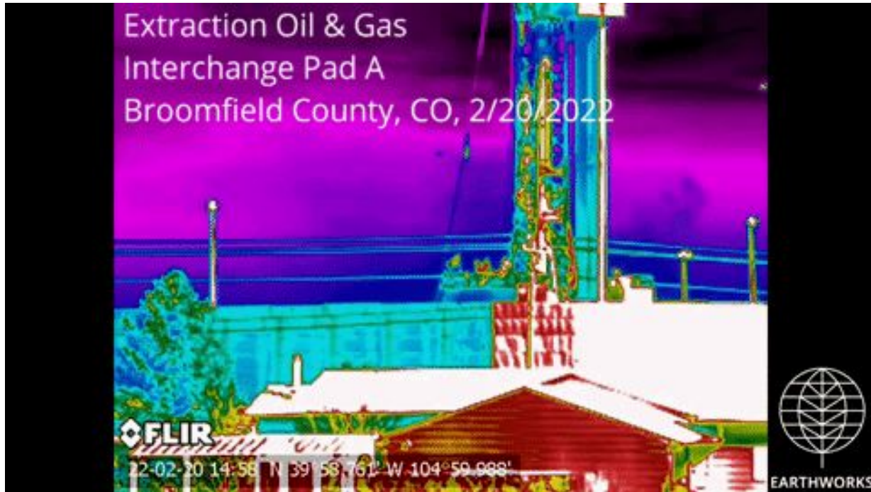
OGI video from same vantage point in early 2022 during drilling phase. Plume of unheated hydrocarbon emissions visible over sound wall
