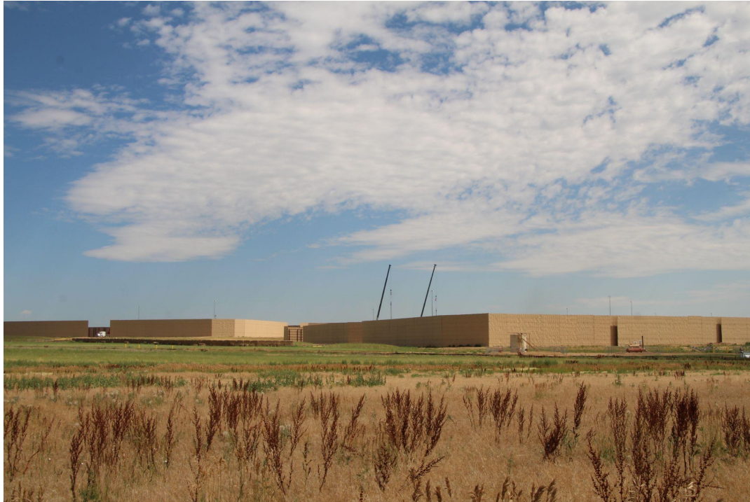
Photo of Extraction Interchange A & B pads from 2019 during pre production.
