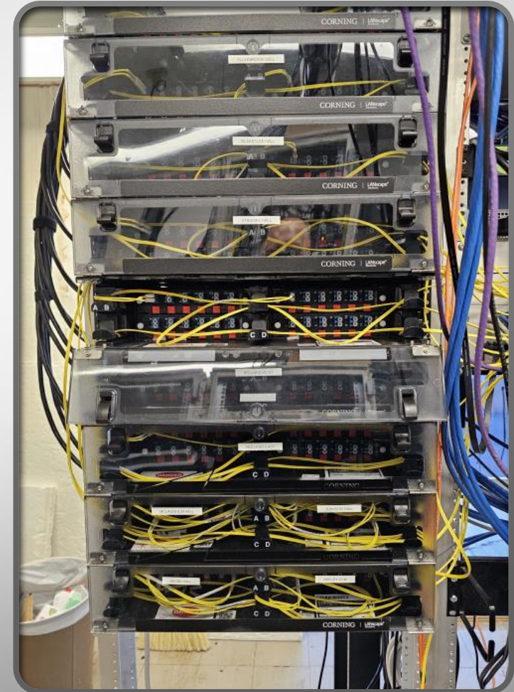
CNCC Data Center – New Fiber Installation
