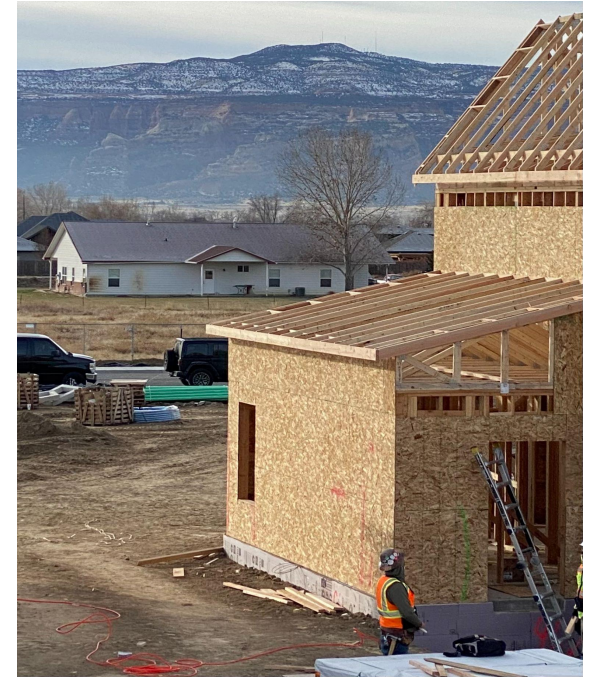
Fruita Mews. Construction of affordable housing units. October 2023.
