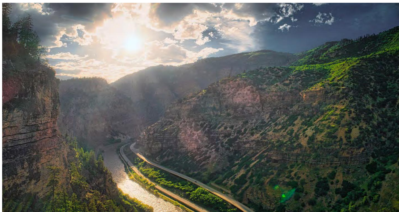
Interstate 70 through Glenwood Canyon Photo Credit: Shutterstock
