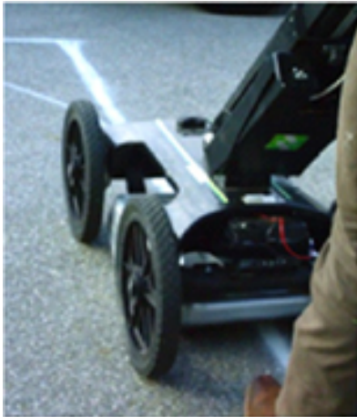
Pre-installation Ground Penetrating Radar
