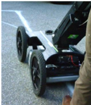
Pre-installation Ground Penetrating Radar
