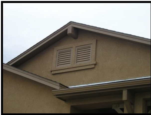
Figure 15 – Example of a gable vent for attic ventilation.
