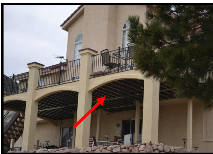
Figure 22 – The arrow depicts the metal floor joists used on this example deck.
