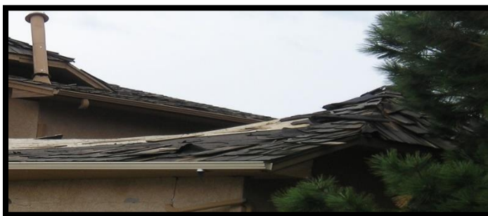
Figure 1 – Example of a shake shingle roof that was ignited from an ember in the 2012 Waldo Canyon fire.
