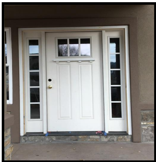
Figure 9 – Example of an approved front door with tempered glass.
