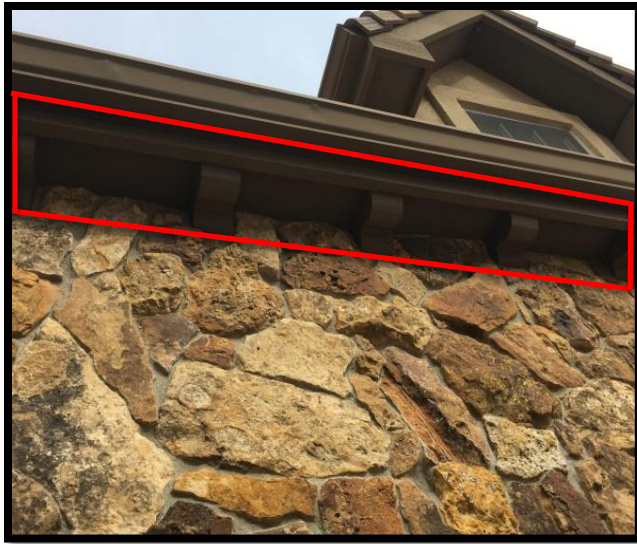
Figure 7 – Example of a corbel on a home
