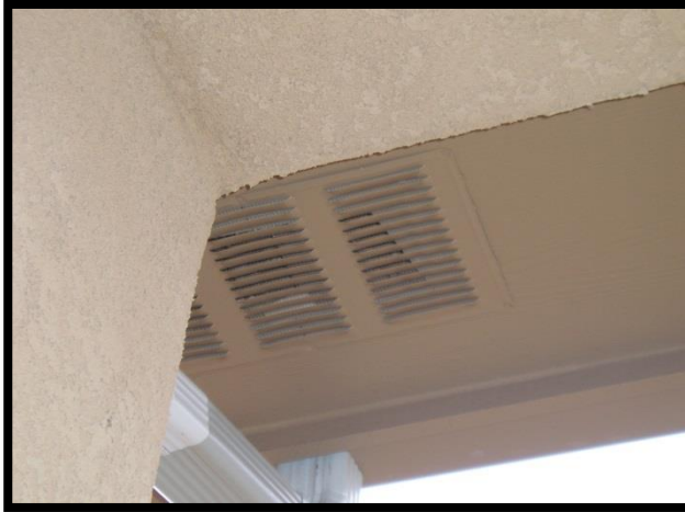
Figure 12 – Example of a soffit vent.
