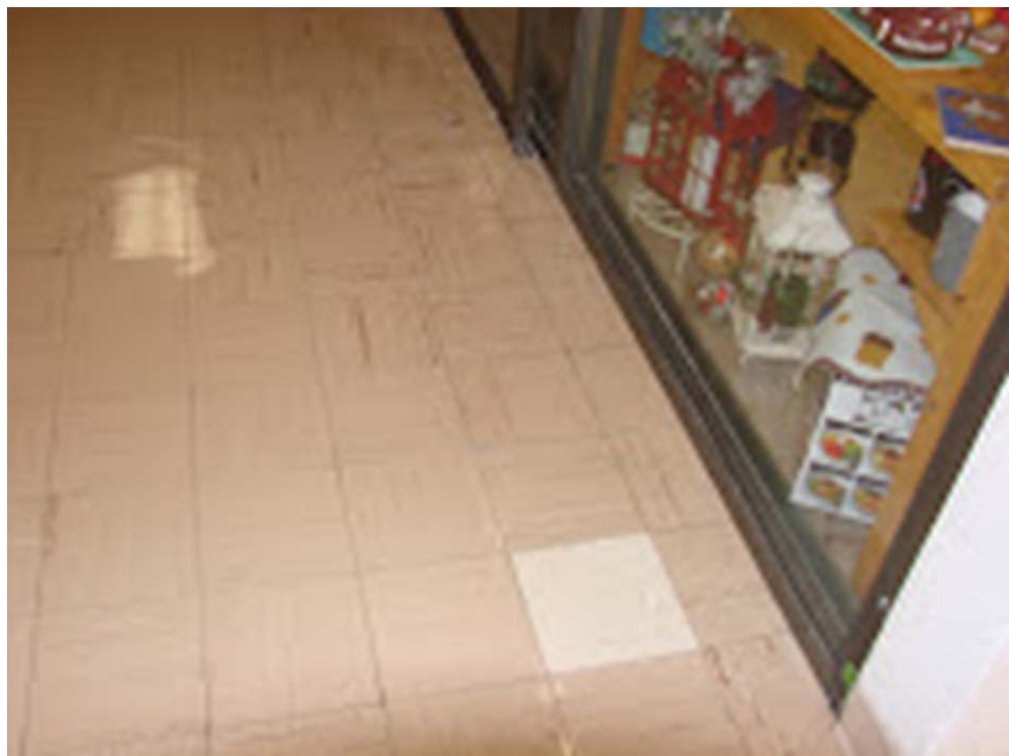
Building A: Mismatched floor tile repair
