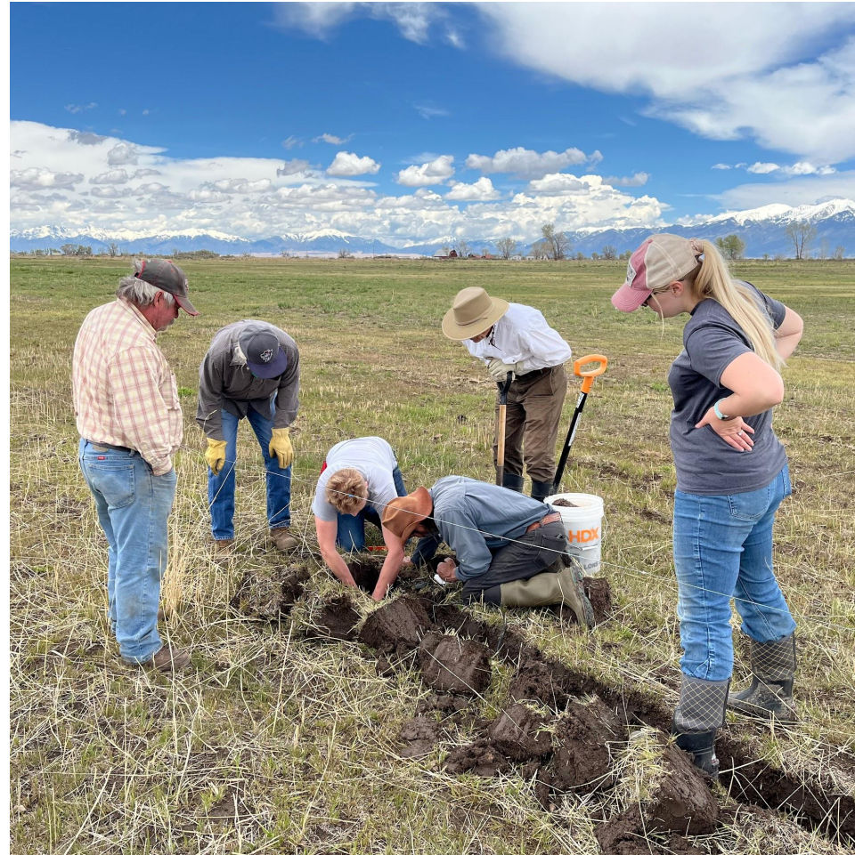
CDA Soil Specialist demonstrates how to install soil moisture monitoring system
