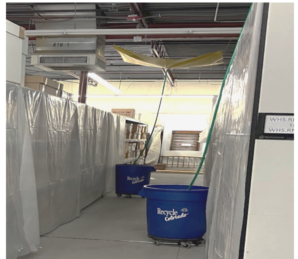
The failing roof often leaks, requiring emergency mitigation to prevent damage to the collections, including tarping and other measures.
