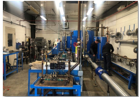
Water meter inspection. Photo Credit: OSA Staff
