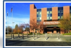
Poudre Valley Hospital
