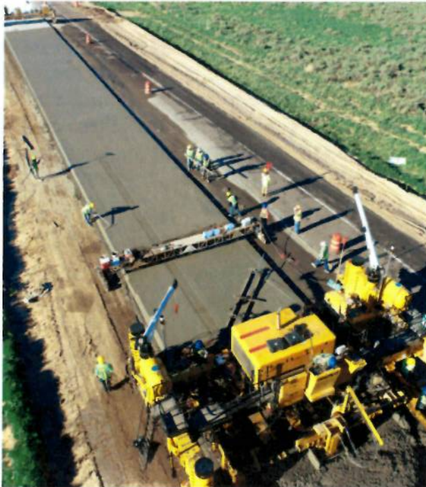
Construction on US 287 in Lamar.
