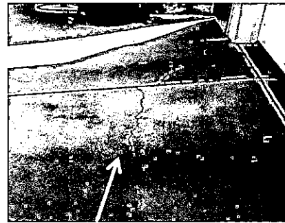
Caused by truck weight and foundation movement. Vibrations from the Extraction Oil & Gas Kennedy/Trott pad resurrections.
