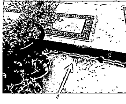
Caused by truck weight and foundation movement. Vibrations from the Extraction Oil & Gas Kennedy/Trott pad resurrections.
