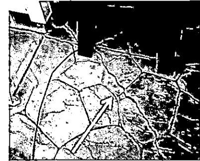
Caused by truck weight and foundation movement. Vibrations from the Extraction Oil & Gas Kennedy/Trott pad resurrections.
