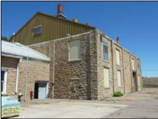
Figure 16: Parcel D – Boiler Plant Exterior
