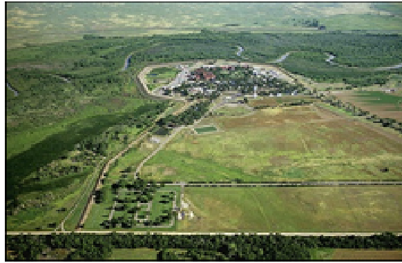
Figure 19: Aerial View of Site – Facing South
