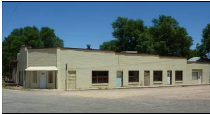
Figure 18: View Northeast from Site Entrance – Abandoned Retail
