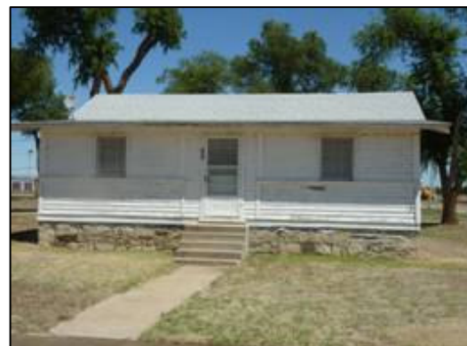
Figure 9: Parcel B – Single-Story Quarters
