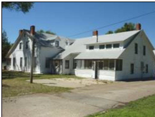
Figure 8: Parcel B – Two-Story Duplex Quarters
