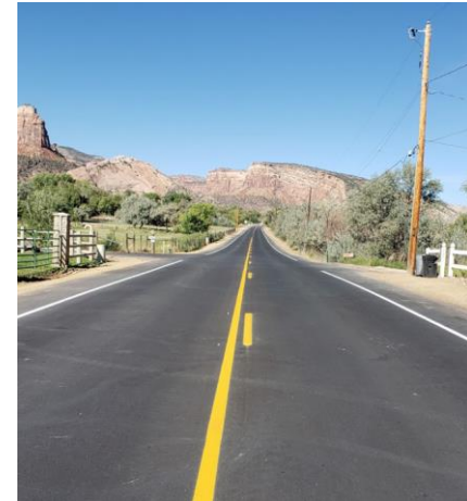
A project on SH340 repaved ¾ mile this summer, including recycling of existing material and adding wider shoulders for safety (August 2020.)
