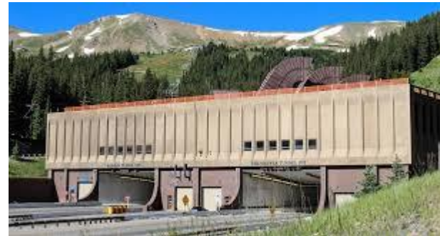
The Eisenhower Johnson Memorial Tunnels.
