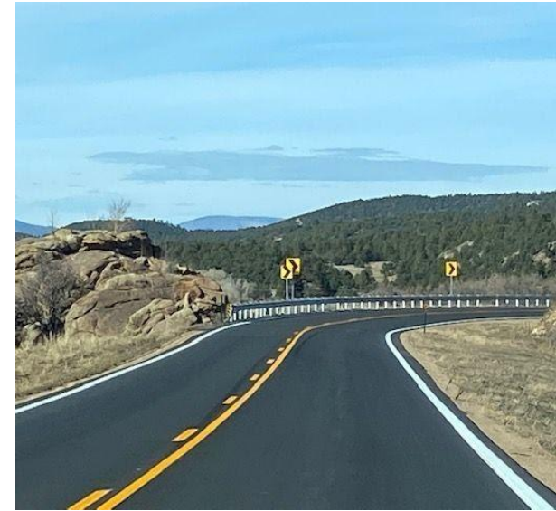
A recent project on CO 69 from Westcliffe to Hillside in Custer County resurfaced almost 13 miles, including critical bridge repairs and safety improvements (December 2020.)
