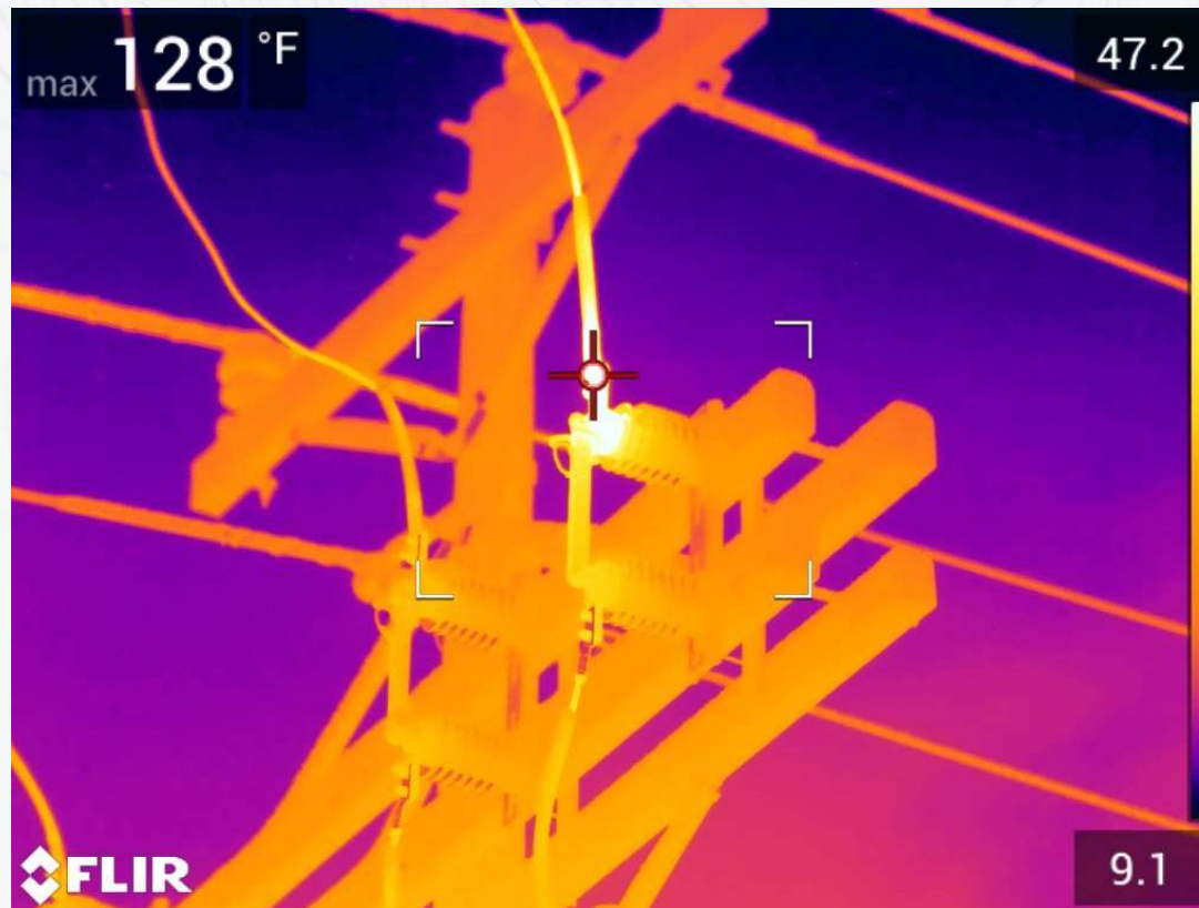
Example Infrared Thermography
